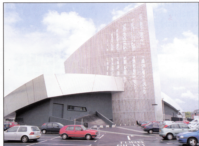
• Ground view external.
